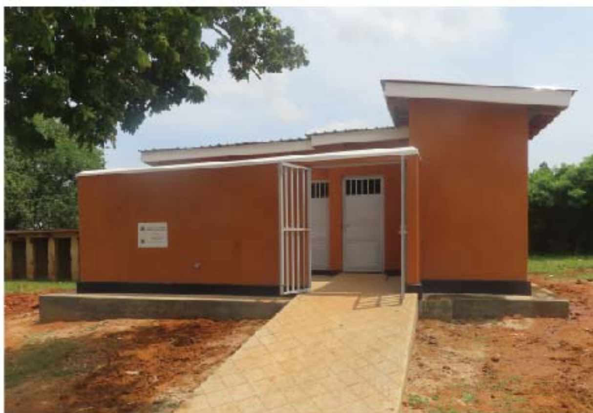
A newly constructed VIP pit-latrine at Siabona P.S in Banda Sub County.
