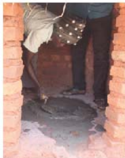
Makhoha using cement to re-enforce a Pit-latrine slab
